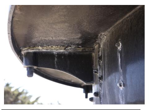
Note missing nut on far right support bracket. Note build up of aluminum oxide along top edge of bracket along seams and connector bolt heads.
