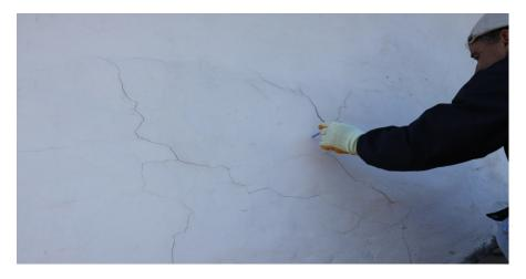
Figure 4: Example of failed stucco coat with resultant loss of protection and additional moisture entry behind stucco coat.
