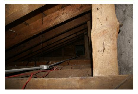
The small crawl space above the kitchen and bathroom area was inspected for indications of roof failure and leaks. Structural integrity and possible wood rot and insect damage were also concerns. No significant damage or any evidence of recent water entry was observed. The wiring system was noted to be in need of inspection and updating to provide adequate and safe electrical service to the lighthouse.
