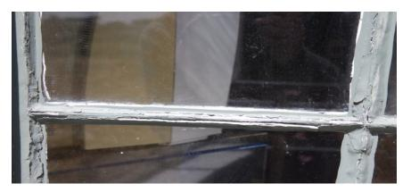
Figure #29: LOSS OF WINDOW GLAZING-POOR
