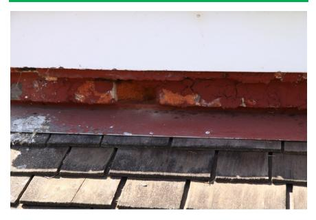
Figure #40: TYPICAL CONDITION OF BRICK CORBEL-POOR.
