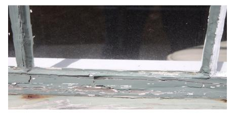
Figure #31: LOSS OF PROTECTIVE COATINGS WINDOW SASH-POOR
