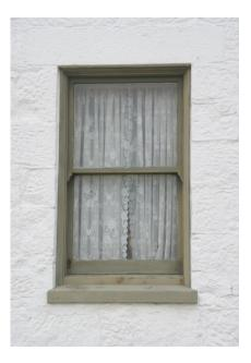
Figure #10: WEST ELEVATION-WINDOW- FAIR to POOR.
