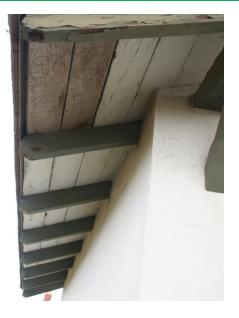
Figure#53: Example of roof deck plank which has been installed to replace damaged historic fabric.
