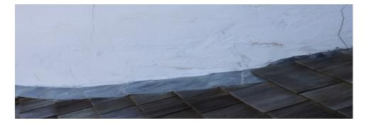
Figure 5: Example of failed stucco coat with resultant loss of protection and additional moisture entry behind stucco coat. Crack allows avenue for water behind metal flashing and into interior walls.
