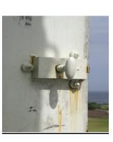
Figure# 11 & #12: Historic lock mechanism must be preserved and used.
