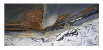
Figure: Damage to deck plate and aluminum flashing.
