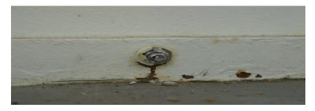
Figure # 9: Stainless steel fasteners used to attach exterior flashing.
