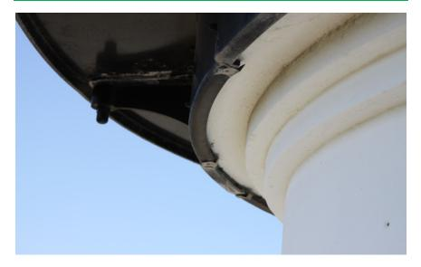
Figure 9: Brick corbel serves as part of lantern room support system.
