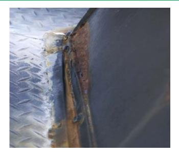
Figure: Base of Lantern Room wall as it connects to deck plate.
