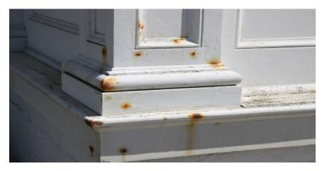
There is a high degree of decorative fenestration on the front porch of the lighthouse. The fenestration has been rated as FAIR to POOR. There is widespread oxidation stains and loss of protective coatings. These conditions could be repaired by volunteers to reduce City of Pacific Grove cost.
