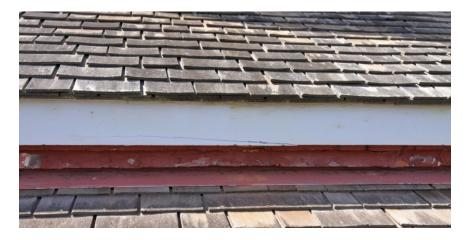
Figure 28: Condition of corbel bricks.
