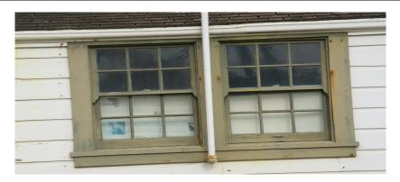
Figure 10: Example of 6/6 double hung **sash** windows- rear attachment.
