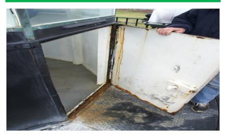
Figure#10: Inside surface of Lantern Room door requires immediate and extensive repair.
