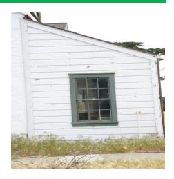
Figure #21: 6/6 DOUBLE HUNG WINDOW -REAR ATTACHMENT-POOR.
