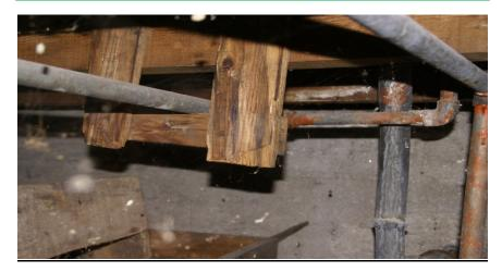
Figure #24: Leaking water pipe below bathroom.
