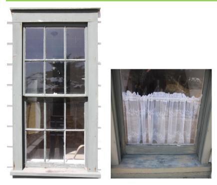
Figure 14 & 15: Example of damage to window trim and window - sill.
