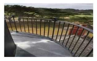
Figure 8: Textured deck plates. Note oxidation of surface.
