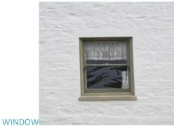
Figure#23 &#24: SOUTH ELEVATION-2<sup>nd</sup> FLOOR WINDOW-FAIR to POOR
