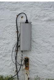
Figure 20 & 21: Obsolete equipment and attachments should be removed and historic fabric repaired.
