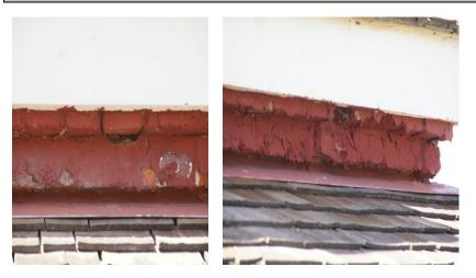
Figure 29 & 30: Examples of type of damage to roof brick corbel.
