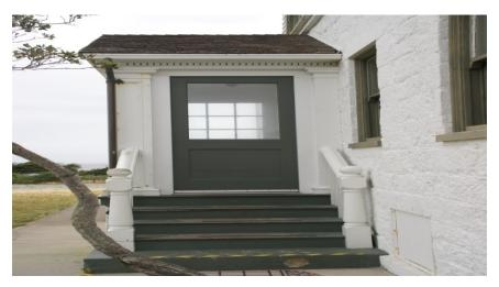
The entrance steps have been rated FAIR to POOR. There are small areas of spaulled concrete requiring patchwork to prevent additional damage and moisture entry.
