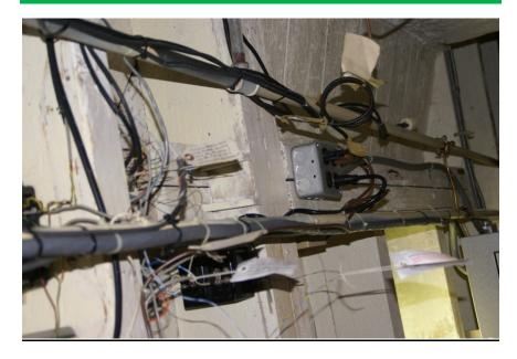
Figure #26 : Maze of electrical lines and conduit in ceiling of basement.
