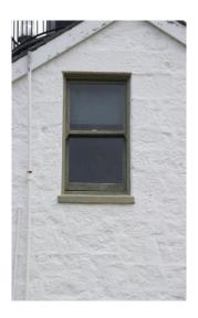
Figure 11& 12: Left and right example of 1<sup>st</sup> and 2<sup>nd</sup> floor 1/1 double hung sash window
