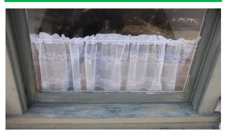
Figure # 30: LOSS OF PROTECTIVE COATINGS -WINDOW SILL-POOR
