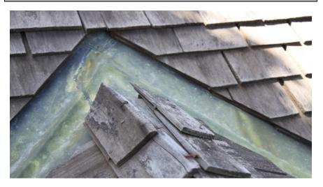
Figure #45 : RIDGE CAP DORMERS-NOTE MISSING RIDGE CAP.
