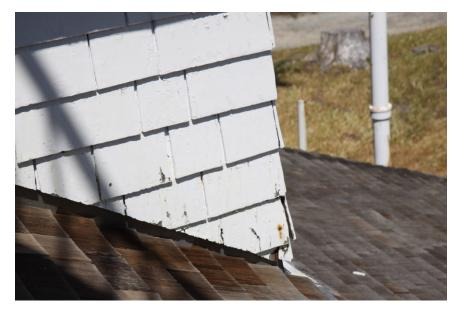
Figure #46: FLASHING AND SHINGLE SIDING DORMERS
