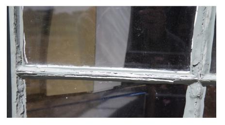
Figure 16: Example of damaged window- pane glazing has loss its integrity and has separated from wooden muntins. Gaps allow moisture between glass and wood fabric.
