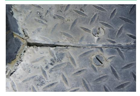
Figure Gallery deck plate-adjoining plate seams.
