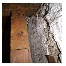
Figure #22: Evidence of earlier plastered wall.
