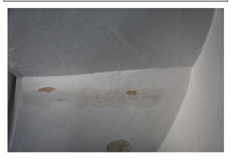
Figure3: Evidence of moisture damage from exterior cracks in stucco.
