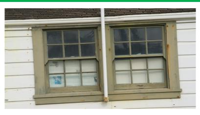
Figure#15 : EAST ELEVATION WINDOWS 6/6 double hung sash windows.-POOR.
