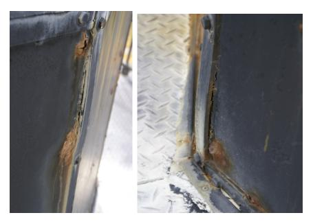
Photo: LR#2 and#3: Loss of integrity of astragals which secure wall panels to lantern room frame.
