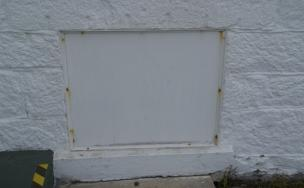
Figure#4 : ENCLOSED BASEMENT WINDOW WEST ELEVATION-POOR.
