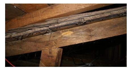
Figure # 21: VIEW OF ATTCI CRAWL SPACE ABOVE ATTACHED KITCHEN AREA. ORIGINAL CEDAR SHAKE SHINGLES FROM PRE-ADDITION WERE STILL IN PLACE.
