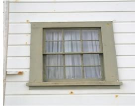
Figure #26 & 27:-ORIGINAL 6/6 DOUBLE HUNG SASH WINDOW-FAIR to POOR.
