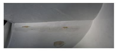
Figure :Moisture stains on inside of lantern support cylinder/stairwell. Conditions Survey: Exterior –Specific Conditions: Page 12 of 55.
