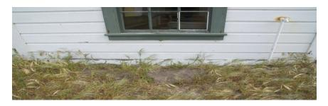
Figure 18: Accumulated dirt and vegetation should be raked away from contact with wood ASAP.
