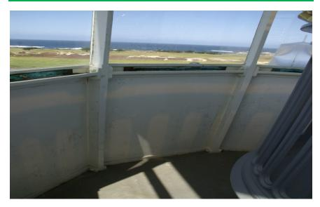
Figure #5: FLAT IRON LANTERN ROOM WALL PANELS.
