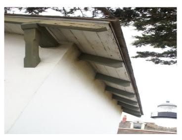
Figure #54: Example of severe crack in fascia board.
