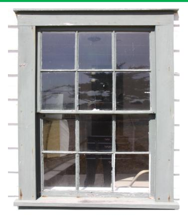
Figure#28 : TYPICAL WINDOW CONDITION-POOR
