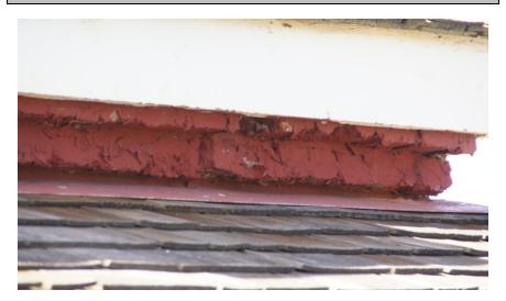
Figure #41: TYPICAL CONDITION OF BRICK CORBEL.POOR
