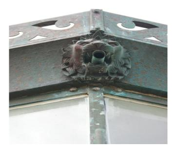
Figure: Bronze Lion Head gutter/downspout
