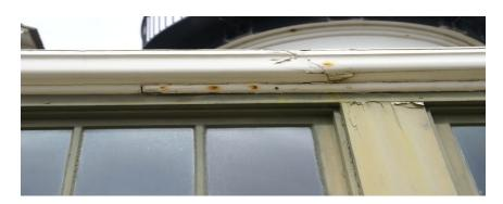
Figure: Gutter system has numerous areas of damage related to failed fasteners.
