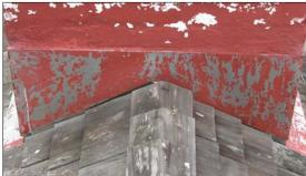
historically inaccurate. The lead flashing at the base of the lantern tower is in good condition; however, cracks were observed at several of the soldered joints that bond together individual pieces.
