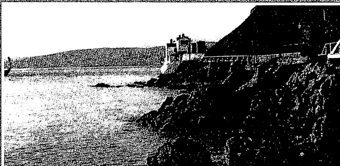
Lime Point Lighthouse and Fog Signal Station as it appeared jutting out into San Francisco Harbor before the Golden Gate Bridge was built. (Photograph courtesy Susan L. Jones Cota.)
