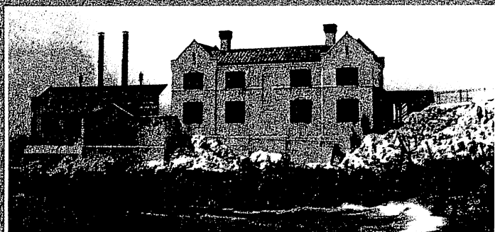
The massive Lime Point Lighthouse and Fog Signal Station near Sausalito, California at the entrance to San Francisco Harbor. Part of the station has since been demolished and the rest of it is now a decaying and forgotten monument to other era. Capt. Peter C. Nelson was stationed here for nearly 30 years. During his tenure the station was in pristine condition. Today, the station is owned by the National Park Service, which has no current plans to save or preserve the structure. (Photograph courtesy National Archives.)
